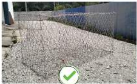
Much better bulging resistant Less bracing wire & efforts
